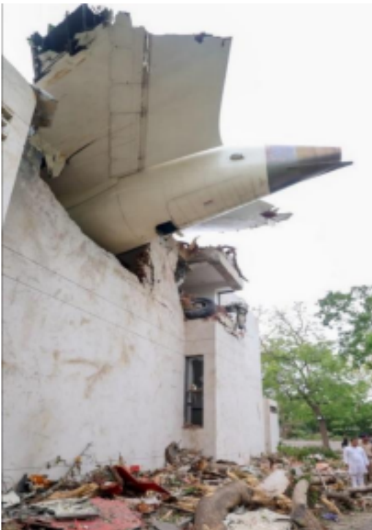
Figure 3 Aircraft attitude at the time of impact with Building A aircraft moved forward, it continued fragmenting and collided with other structures and vegetation. The impact witness marks on the building and airplane indicated a likely nose-up attitude (about 8°) and wings level.
